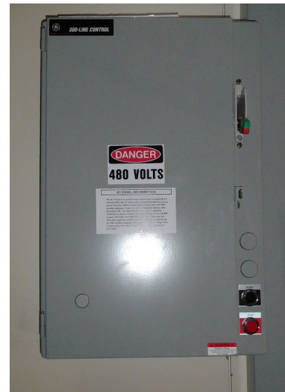
Figure 34: Emergency Shutdown Buttons
