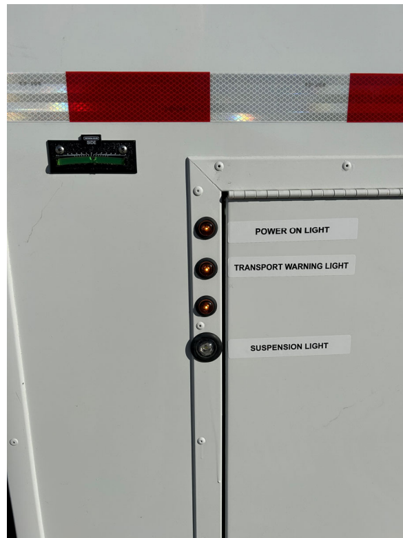
Figure 63: Lift Transport Warning
