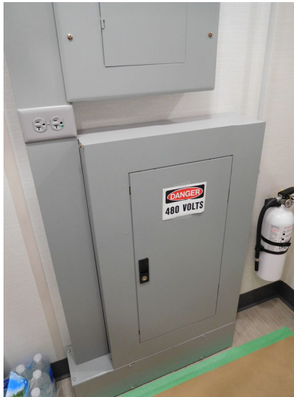
Figure 36: 480V AC Electrical Panel
