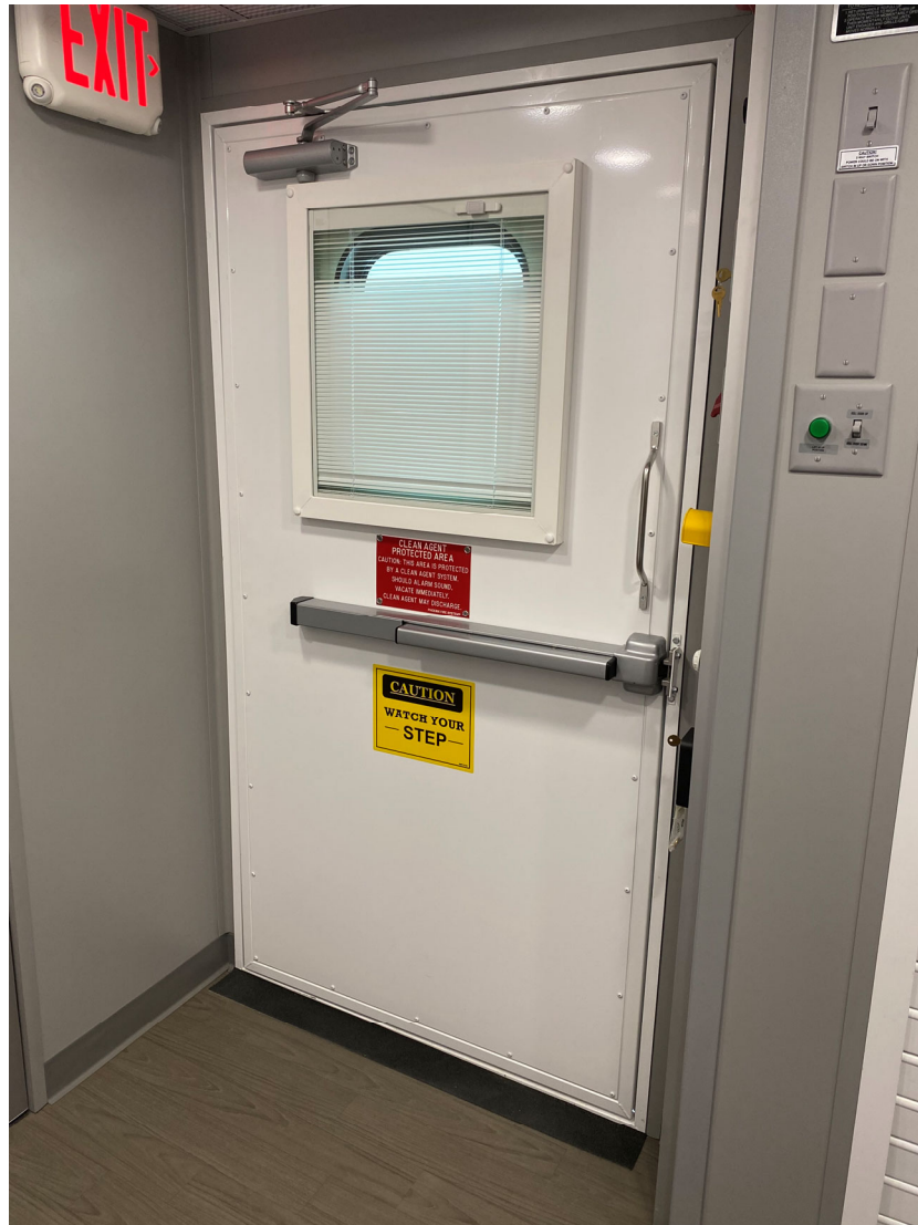
Figure 9: Exterior Staff Door
