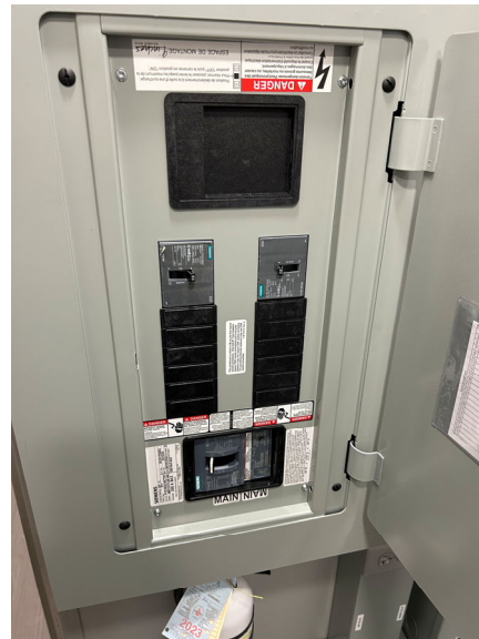
Figure 36: 480V AC Electrical Panel
