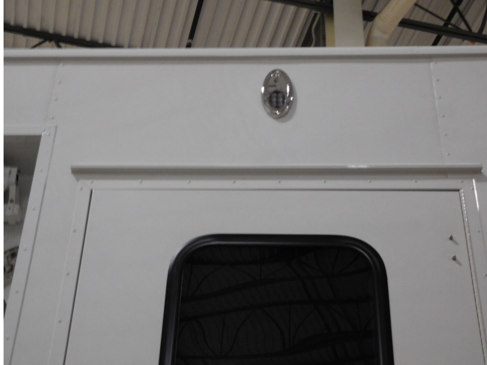
Figure 57: Staff Door Lighting
