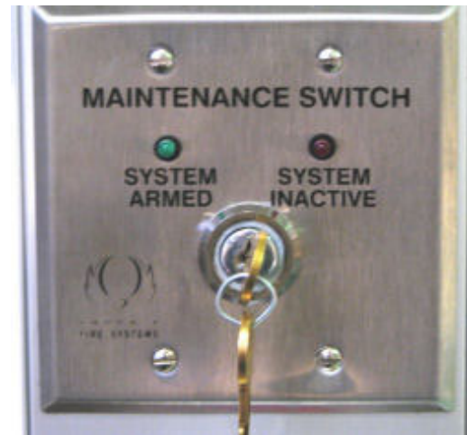
Figure 32: Maintenance Switch
