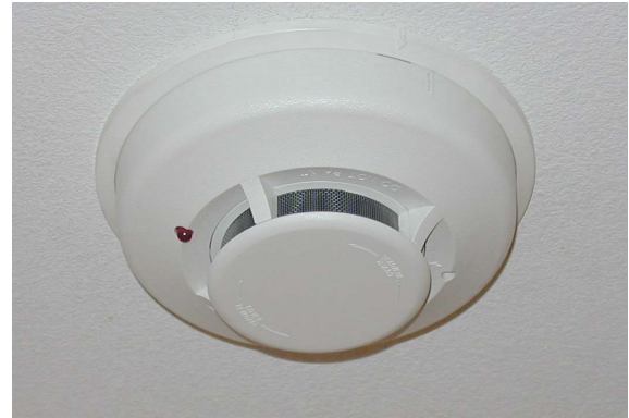
Figure 26: Smoke Detector
