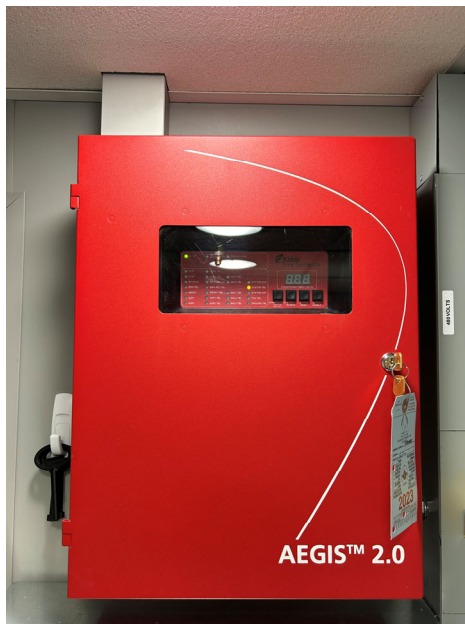
Figure 27: Fire Alarm Control Panel
