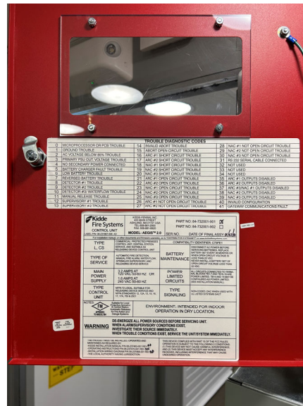
Figure 27: Fire Alarm Control Panel
