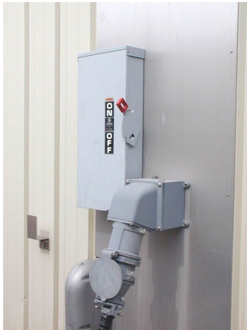
Figure 26: Shore Power Connection
