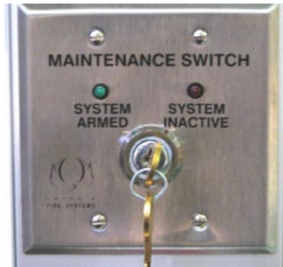
Figure 22: Maintenance Switch
