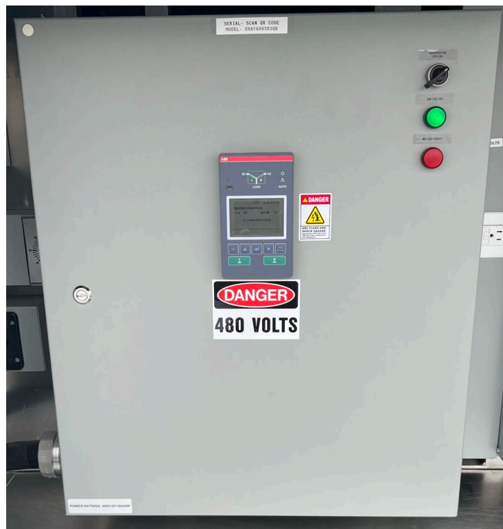
Figure 27: 480V AC ATS and Phase Power Monitor
