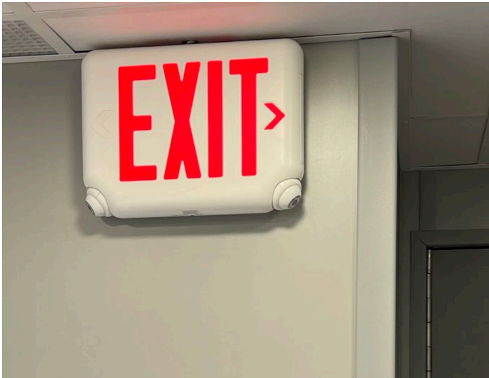
Figure 15: Control Room Emergency Lighting
