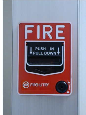
Figure 18: Fire Alarm Pull Station
