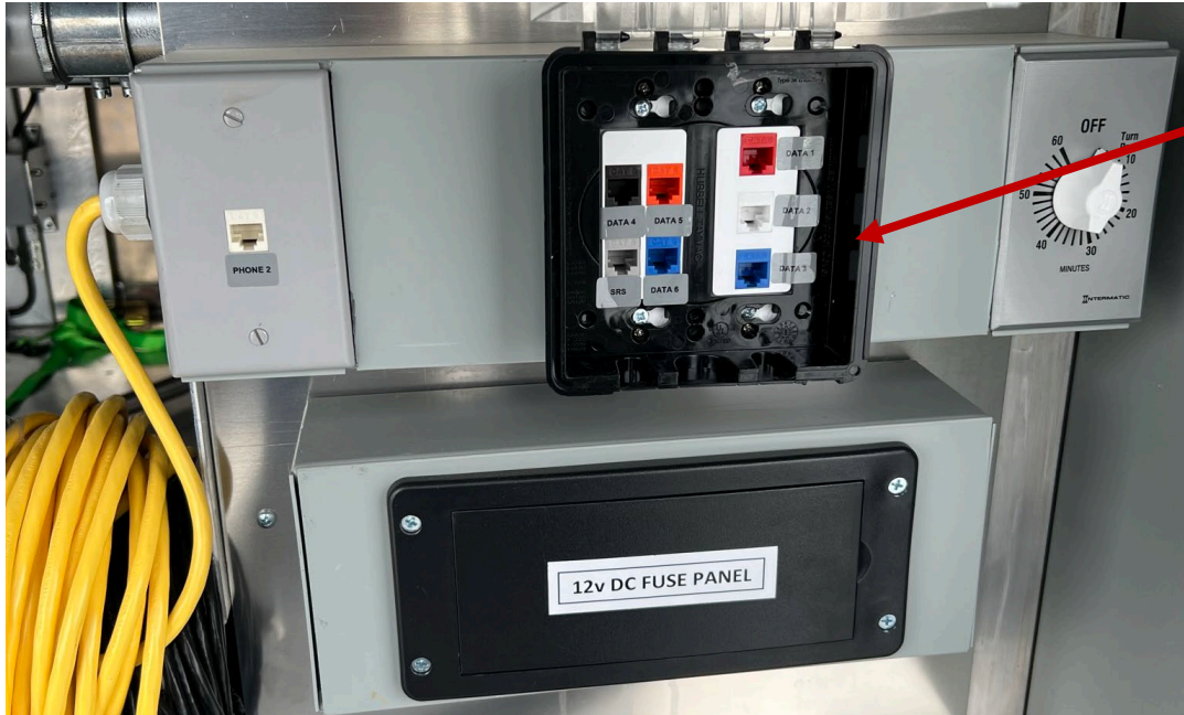
Figure 11: Phone & Data Line Connections
