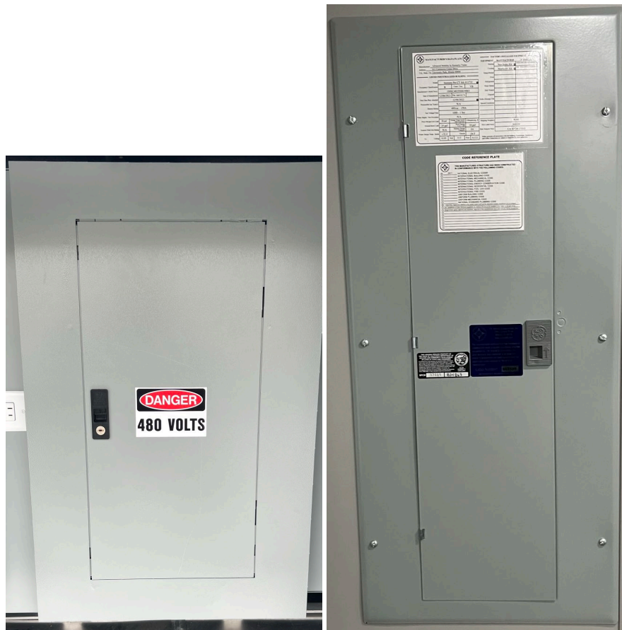
Figure 26: 480V and 120/208V AC Electrical Panels
