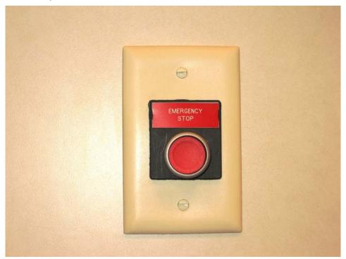
**Figure 5: Emergency Shutdown Buttons**
