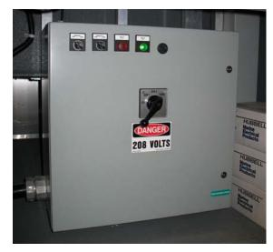
Figure 19: 208V Power Control Panel
